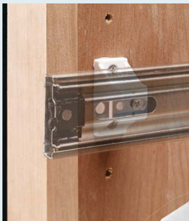
▲ Spacers make it easy to install drawer slides in a face frame cabinet.
