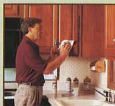
Cabinet Refurbishing - cleaning, degreasing, repairing and polishing
