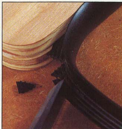
Cut V-notches from the molding's spline to help it bend around radiused corners. A narrow chisel prevents damage to the molding's edges.
